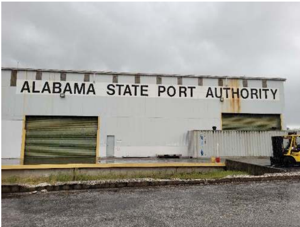
West Side of Pier 3 Warehouse
