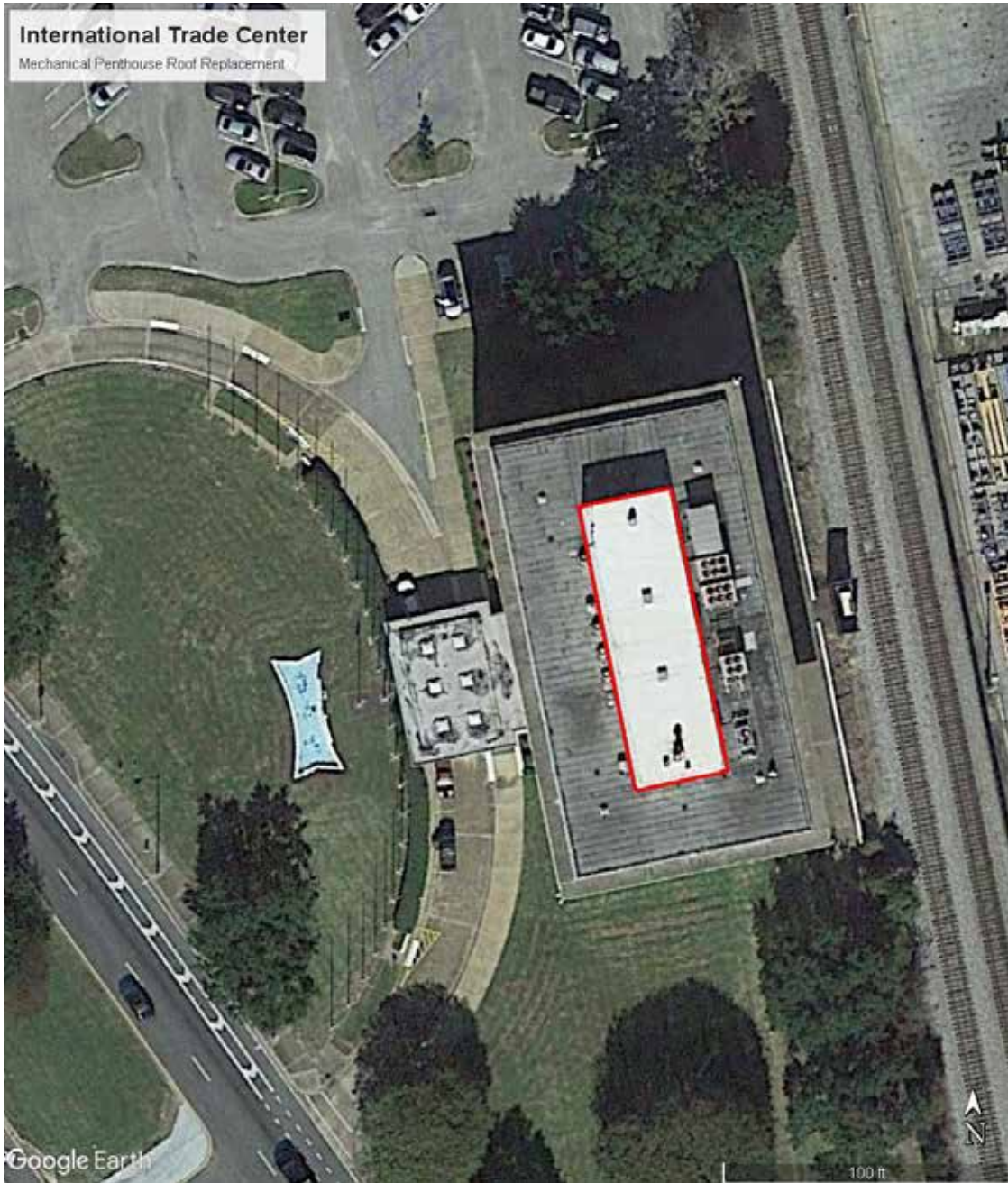
Penthouse Roof Outlined in Red – Approximately 3,100 square feet
