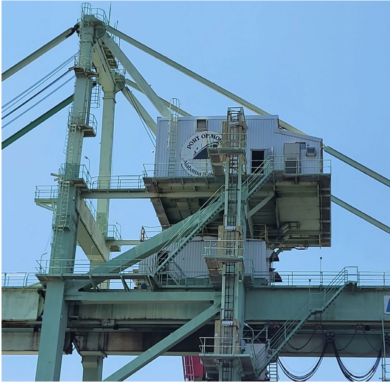
M Crane on Dock 3 – Looking South
