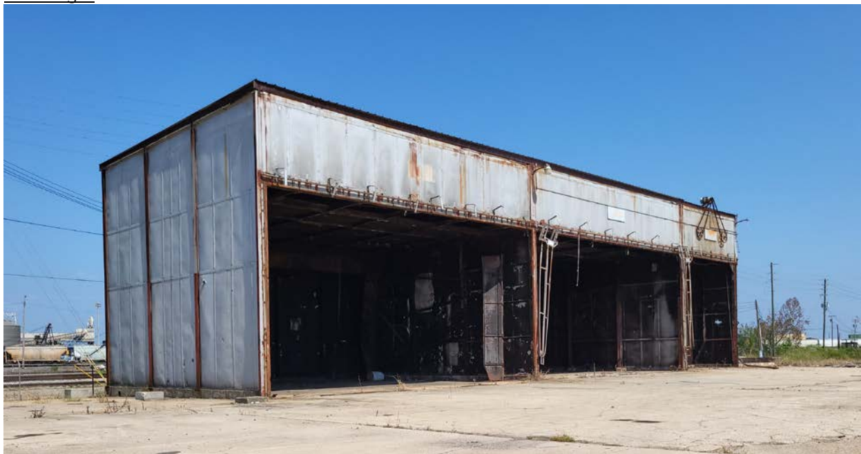
Building 7 – To be demolished
