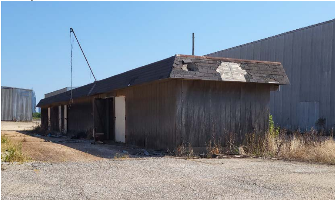
Building 1 – To be demolished
