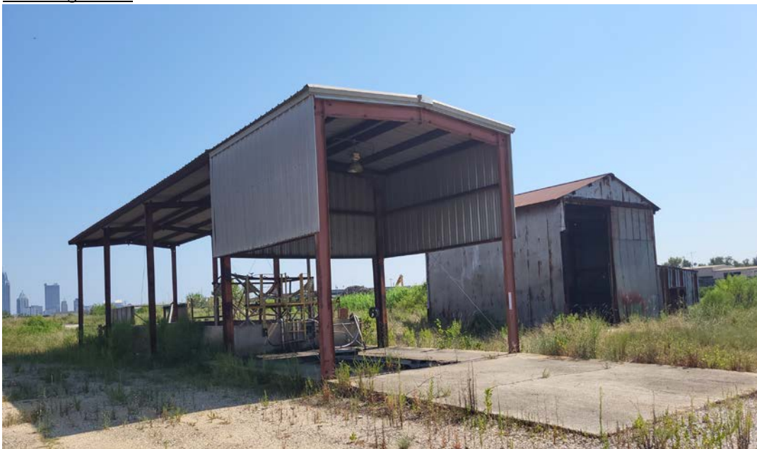
Building 2 & 3 – To be demolished
