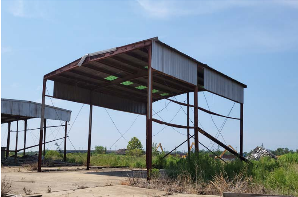
Building 4 – To be demolished
