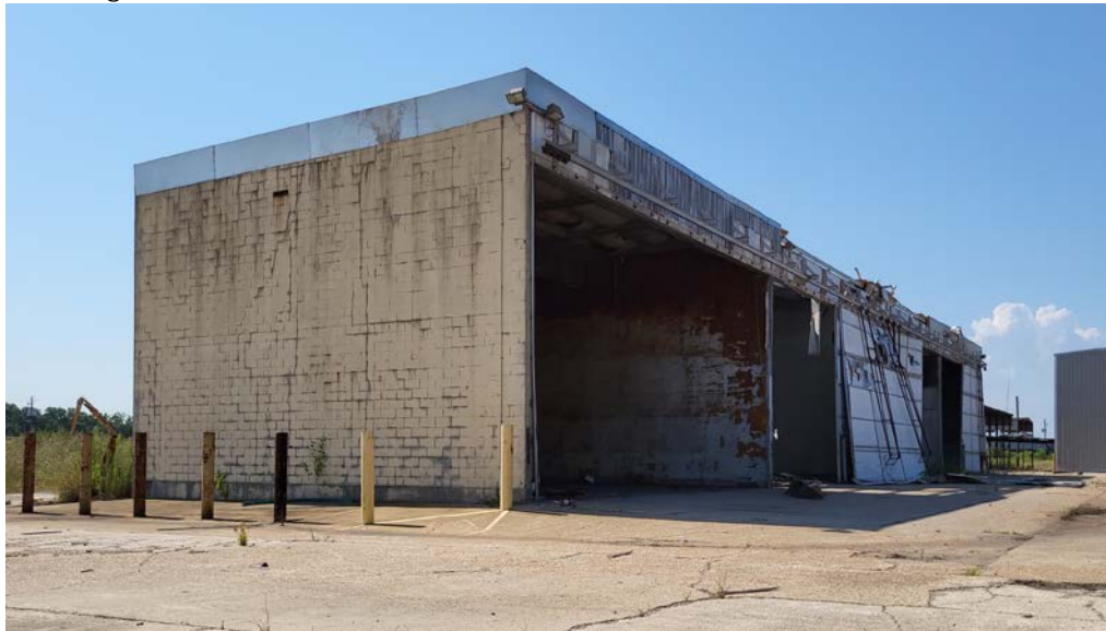
Building 6 – To be demolished
