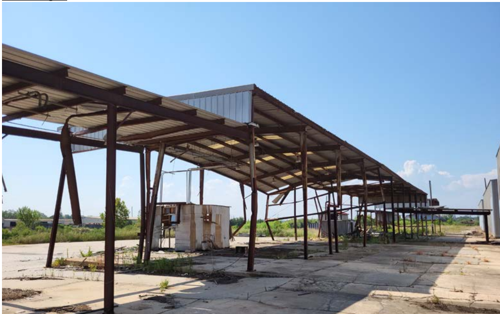
Building 5 – To be demolished
