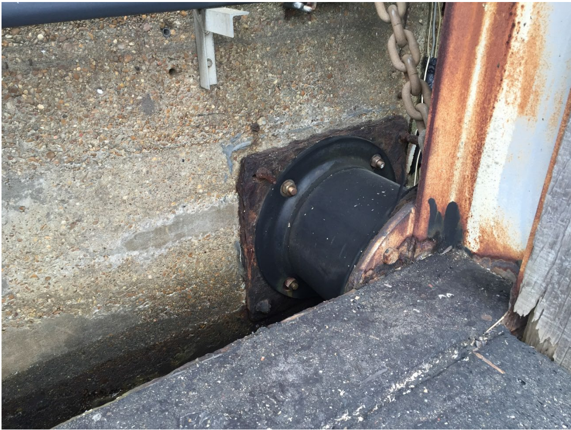
Typical Berth 2 Fender System – Looking West
