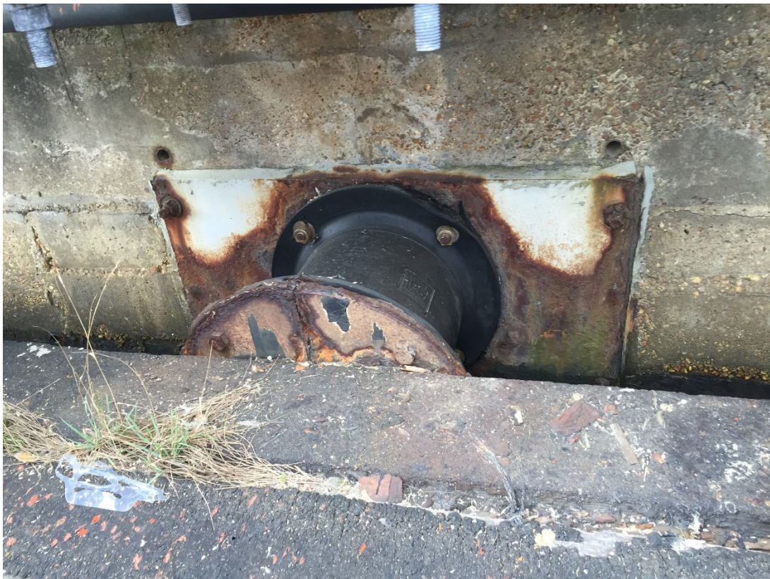
Typical Berth 2 Fender System – Looking West
