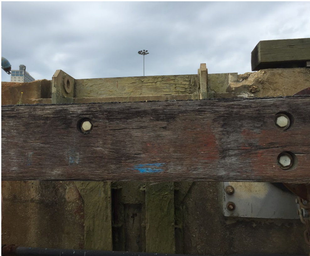
Typical Berth 2 Fender System – Looking West
