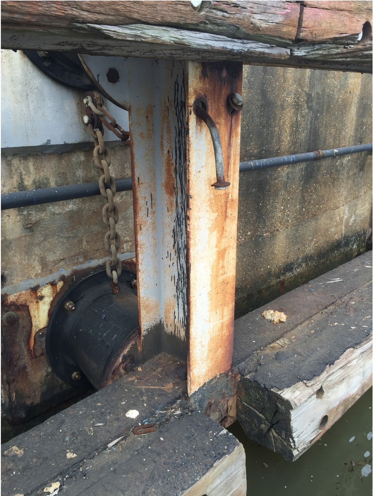
Typical Berth 2 Fender System
