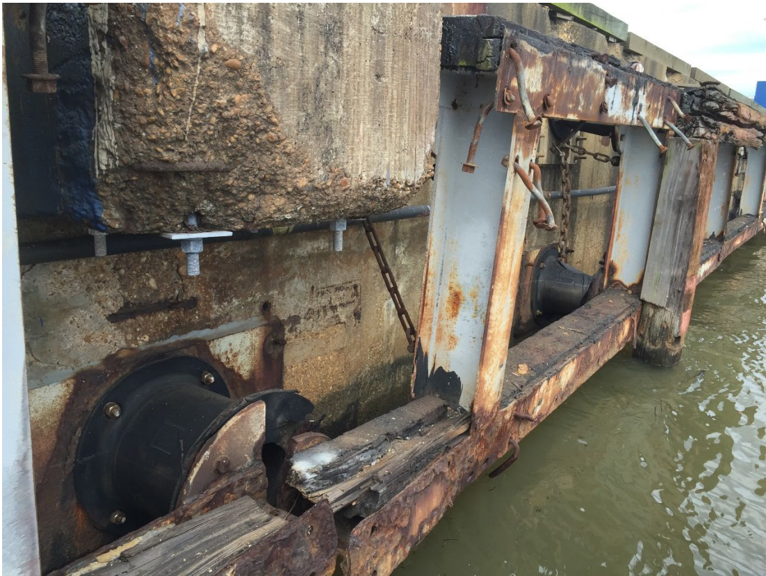
Typical Berth 2 Fender System – Looking Northwest
