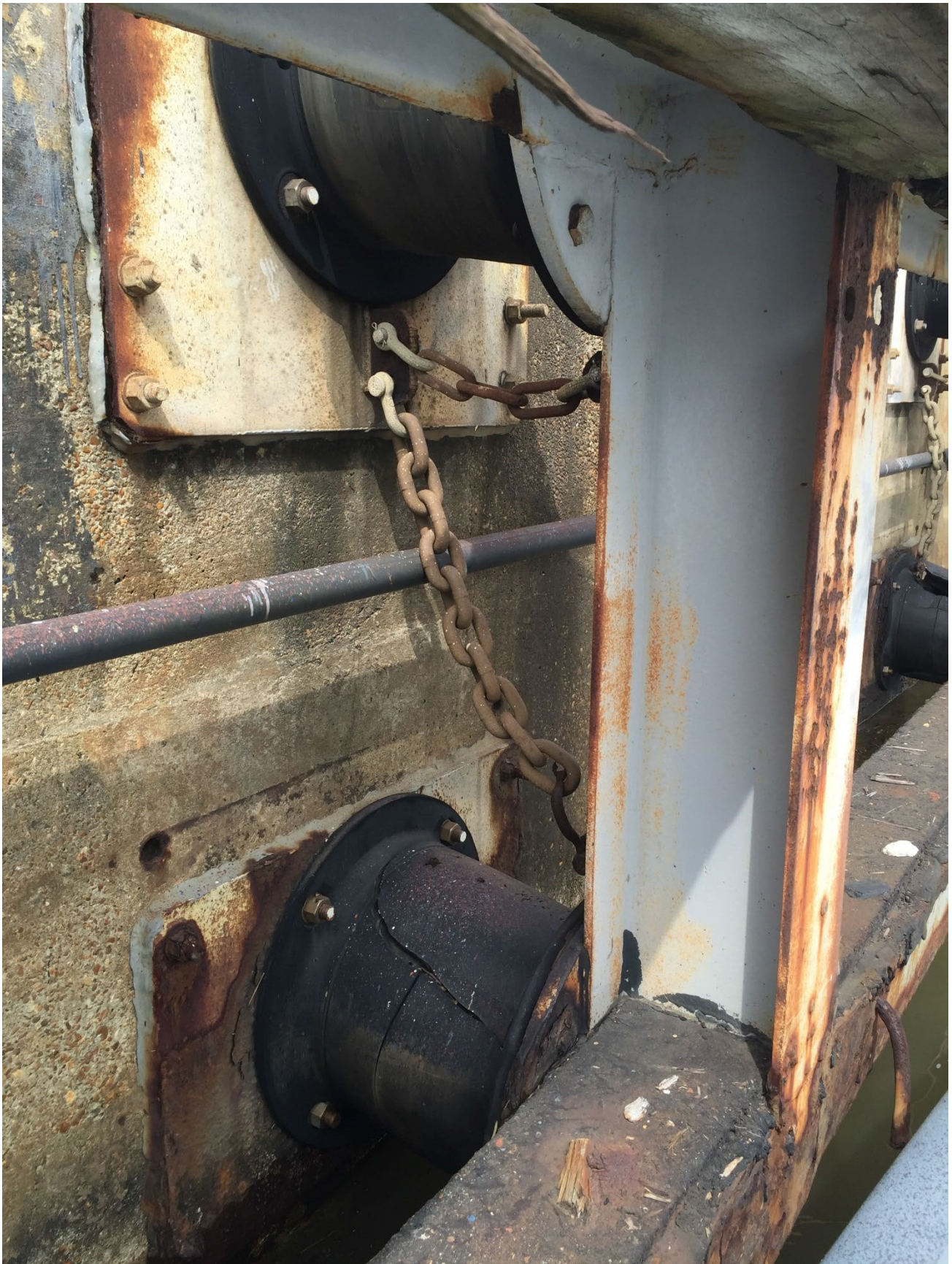
Typical Berth 2 Fender System
