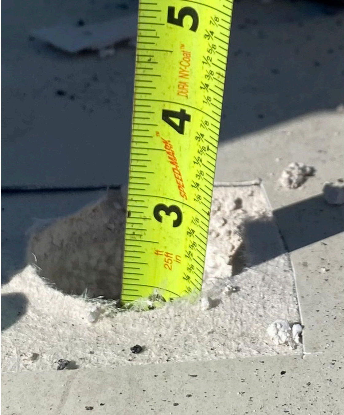
Roof System Thickness at Sample 1 and 3 (See drawing for sample locations)
