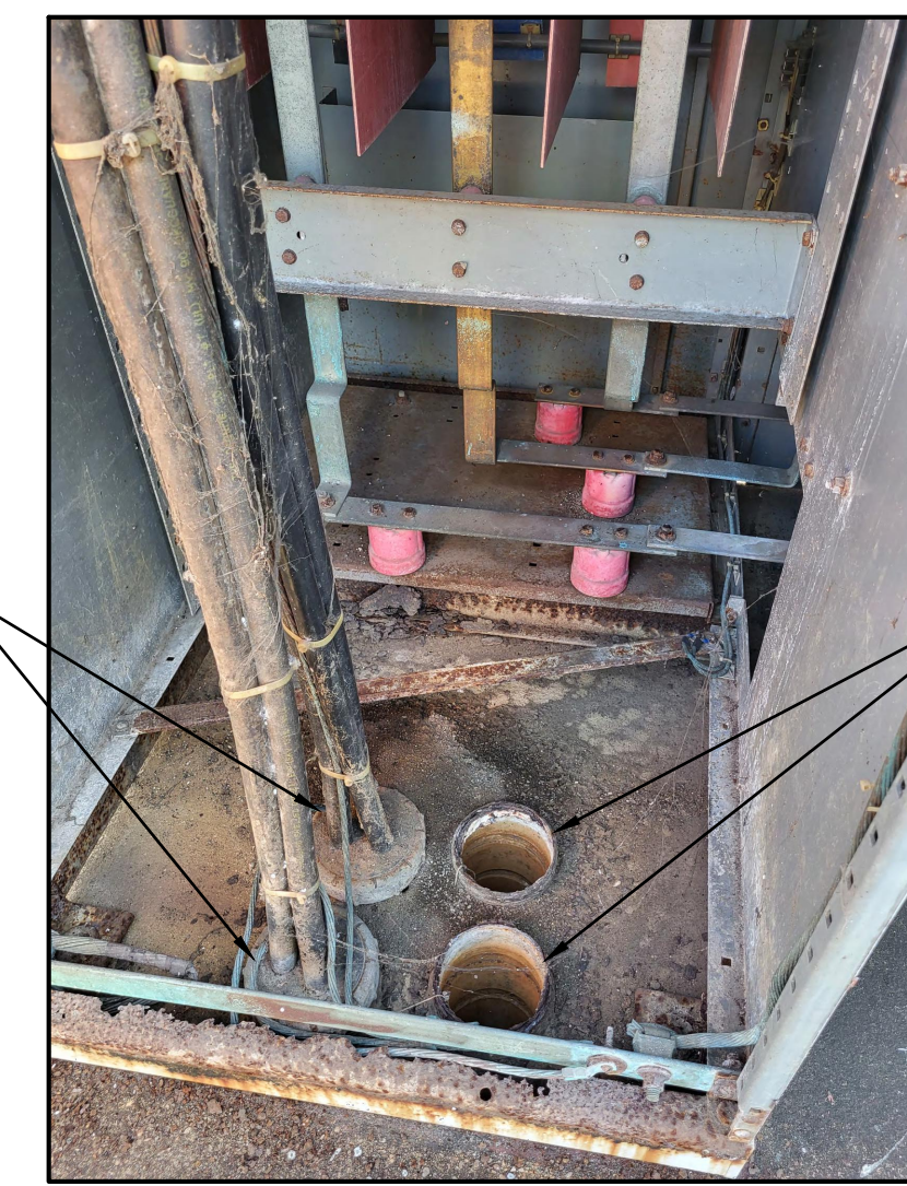
2 EXISTING CONDUIT PENETRATIONS MAIN MEDIUM VOLTAGE SWITCH NOT TO SCALE
