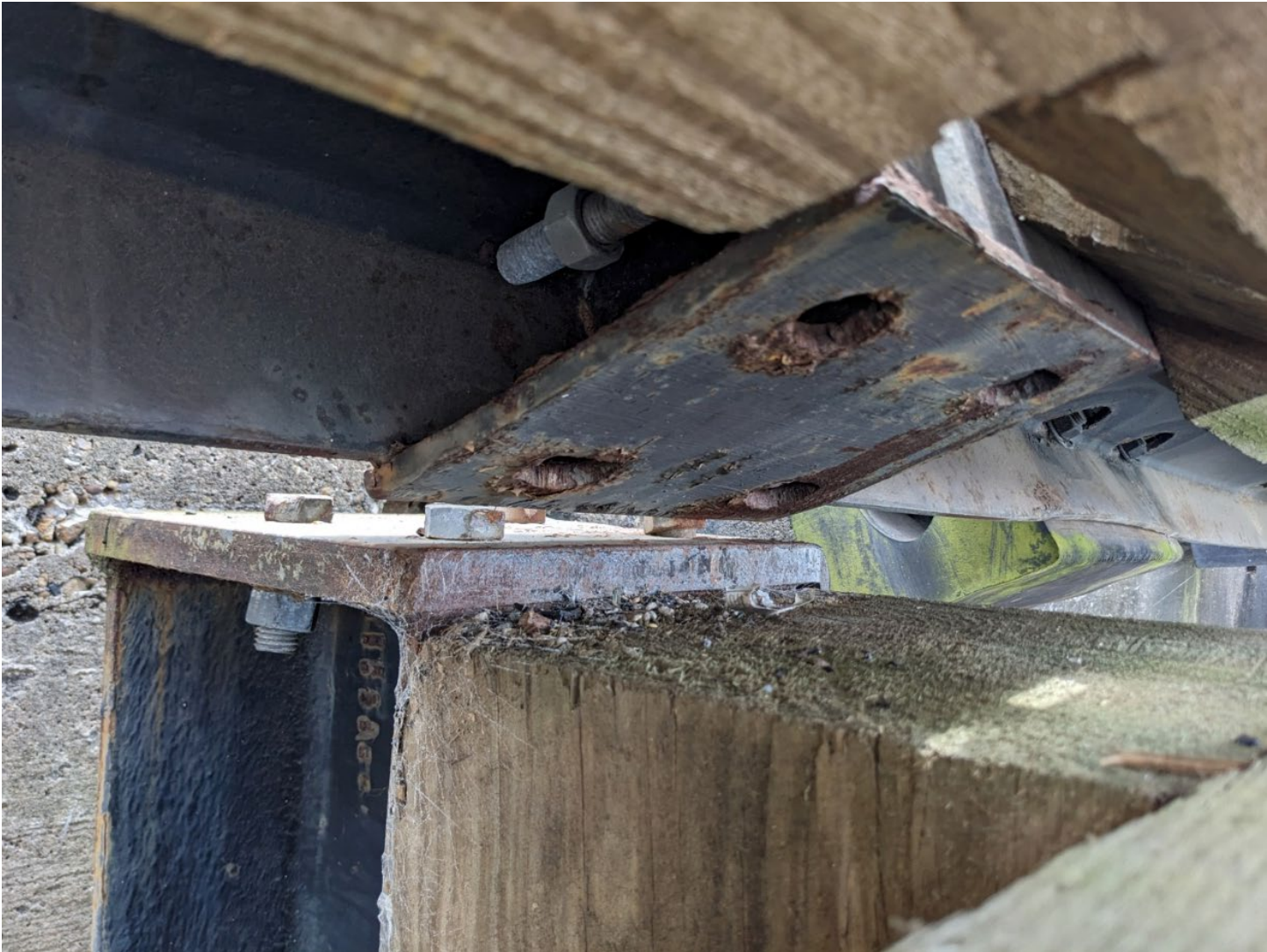
Plate connection for horizontal steel wale to vertical pile
