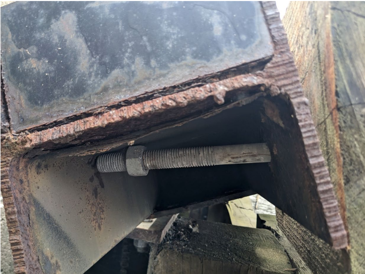
Side view of steel wale
