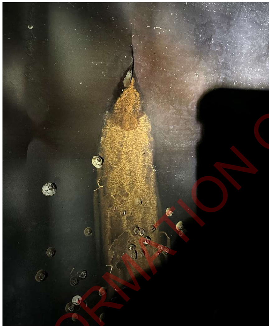
Typical Minor Hairline Crack in Inner Lining of Pipe
